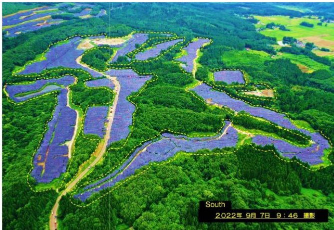
Figure 1: Onikoube's construction nears completion
